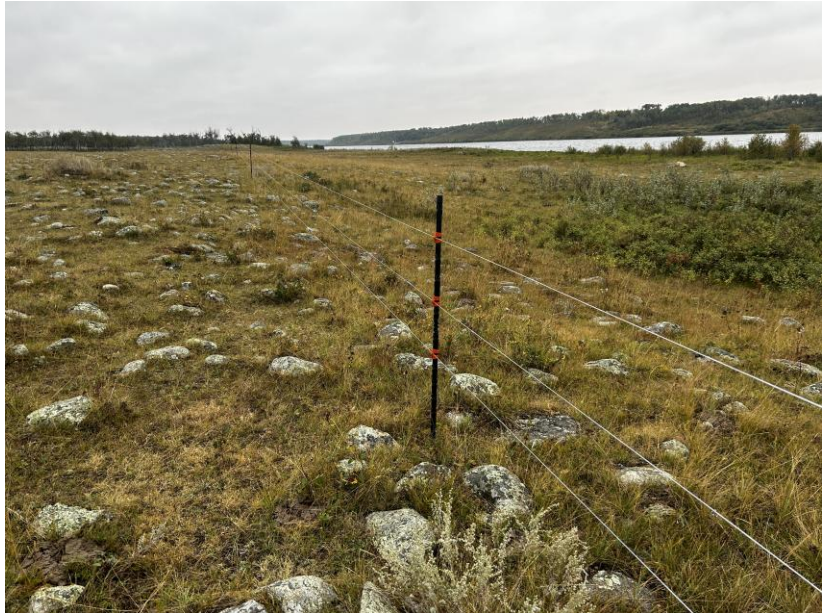
3-strand electric high tensile fencing with Gallagher plastic posts proved the only feasible option for fencing the extremely rocky shoreline.
