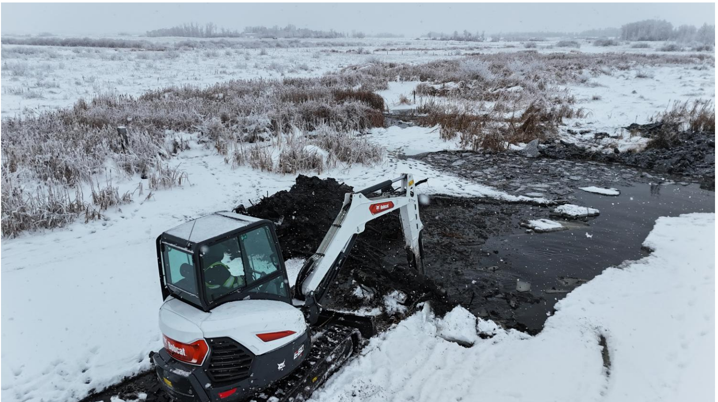
November 2024: Removal of Secondary Dam
