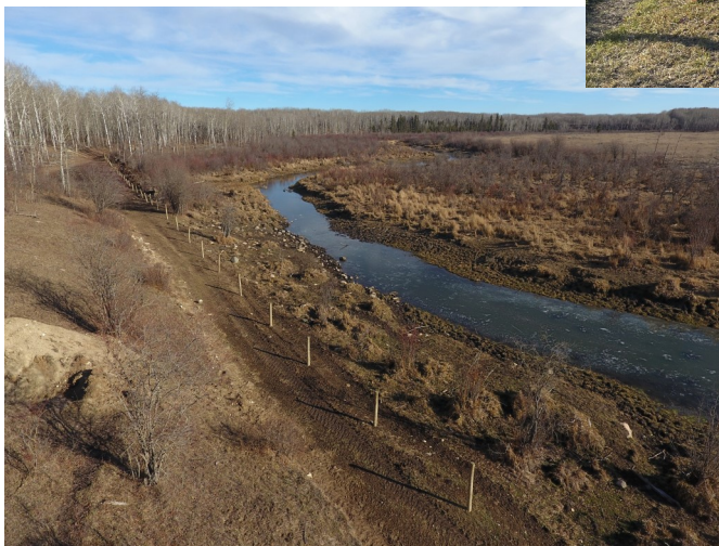
Permanent 4-strand barbed wire fencing installed along the Assiniboine River
