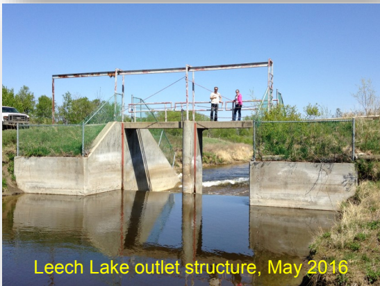
Control culvert on YCWAB-sanctioned ditch
