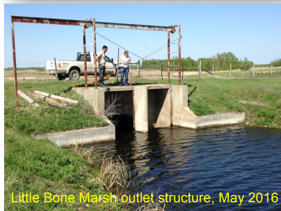
Control culvert on YCWAB-sanctioned ditch
