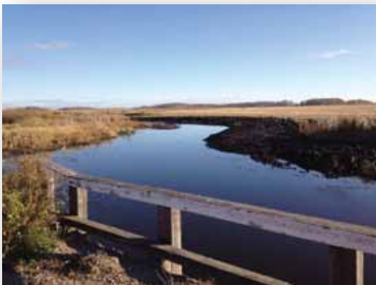
Channel Clearing - "Sleepy's Bridge" (Oct.17/14)
