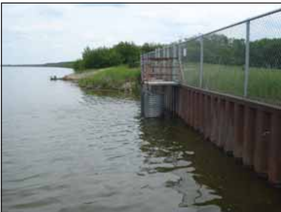
3-culvert outlet structure and overflow spillway in SW corner of Good Spirit Lake
