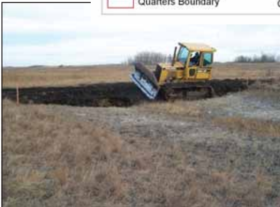
The contractor installing ditch plugs
