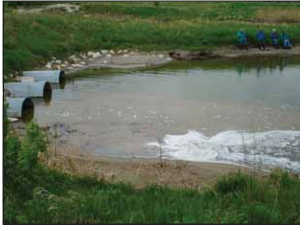
2010 - The culverts are overwhelmed, the lake reached high levels and also ran over the spillway
