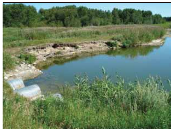
Sept. 2013 - The scour hole just prior to construction
