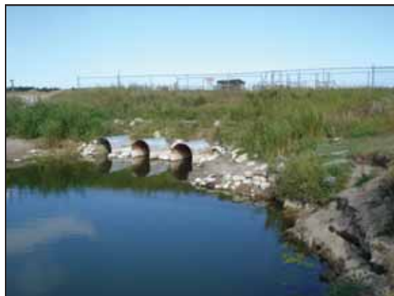
3-culvert outlet structure and overflow spillway in SW corner of Good Spirit Lake
