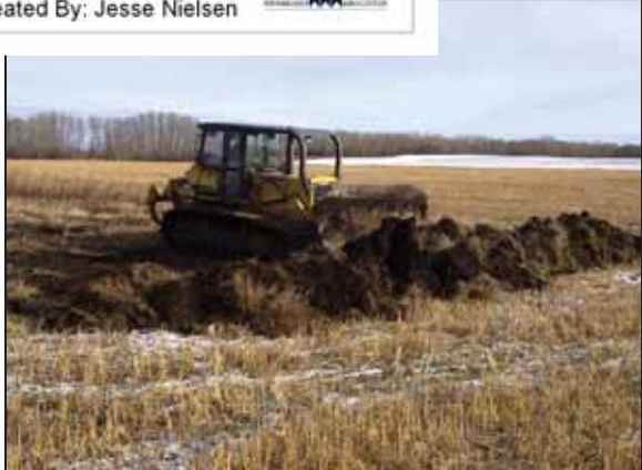
The contractor installing ditch plugs
