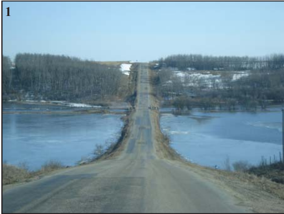
1 April 13 th - Highway #47 North of Springside
