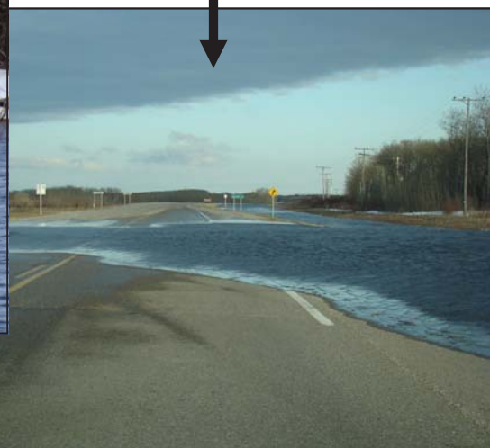
Highway #16 - at Sheho
